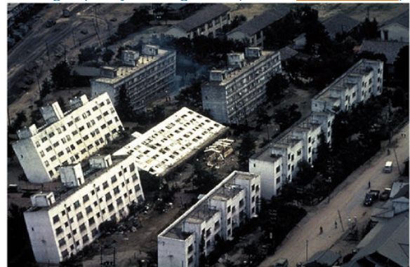
Figure 4. Buildings have toppled due to a loss of the bearing capacity of the ground (Photo: www.nap.edu ).
