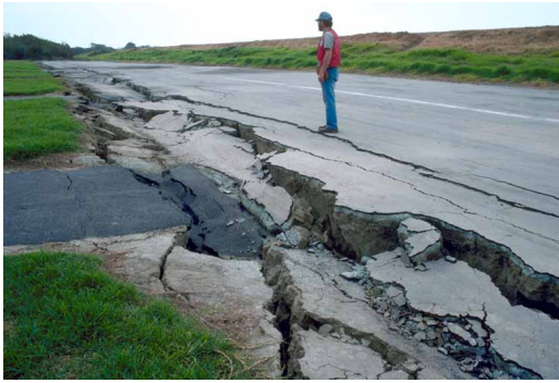
Figure 2. Lateral spreads caused by liquefaction of the soil (Photo: USGS Multimedia Gallery).
