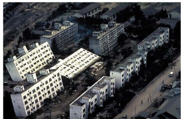
Figure 4. Buildings have toppled due to a loss of the bearing capacity of the ground (Photo: www.nap.edu).
